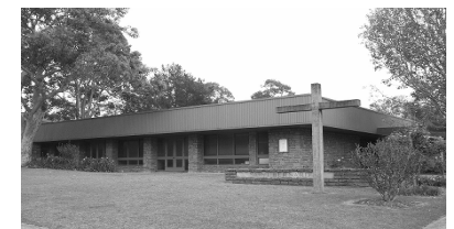
Parish Church of Saint Bernard Berowra Heights
